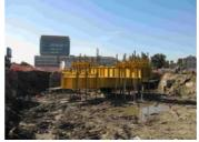
Top down 30 MN Static Load testing reaction system
